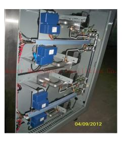
High-quality and durable heating control system Ignitor, air blower and solenoid valve
